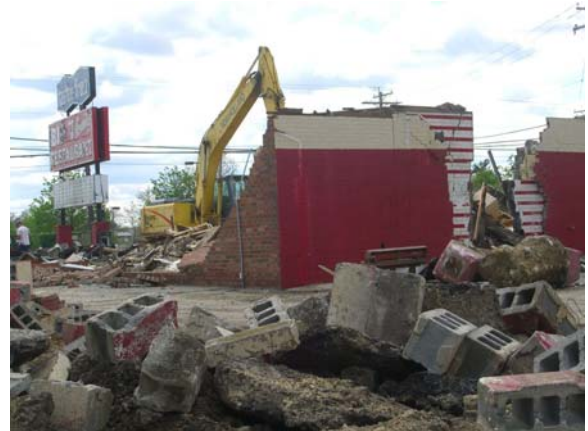
Demolition of Tastee Freeze/McDonald's photograph submitted by Mike McLaughlin
